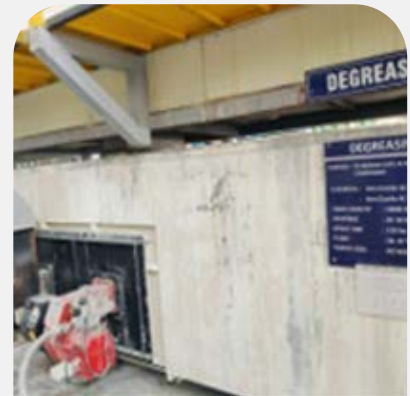
At degreasing (To remove dirt and grease from component)
